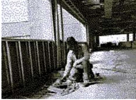
**Electric Winch Used To Lower Panels Over Edge of Slab**
