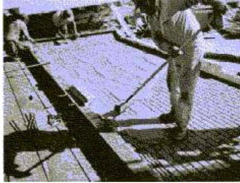
**Grouting Over Back Surface of Thin Brick Panel**
